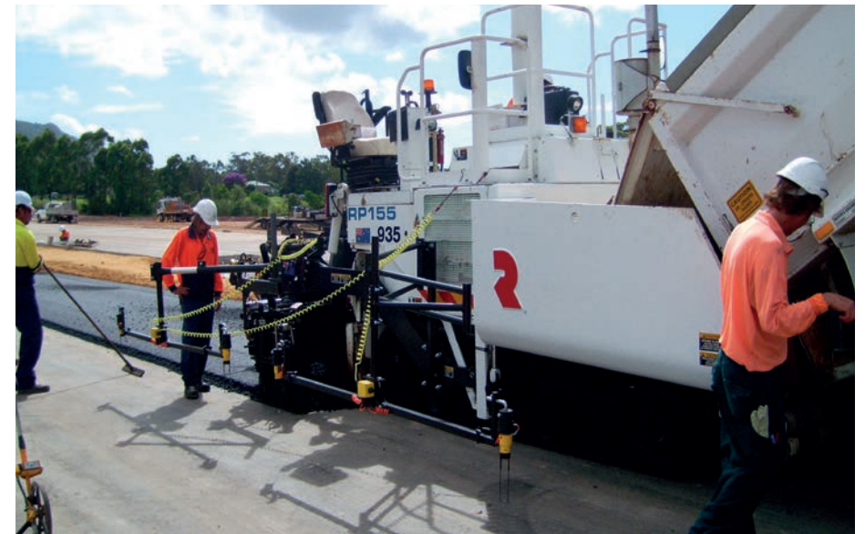
Averaging Beam with four grade sensors.
