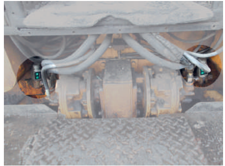
Mounting of AC700 on both conveyor belts
