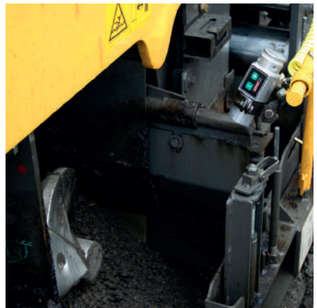
Mounting of the AC700 at the auger
