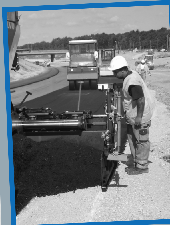
Mini-Line® HS301 Grade Control Kit with G224 on a stringline
