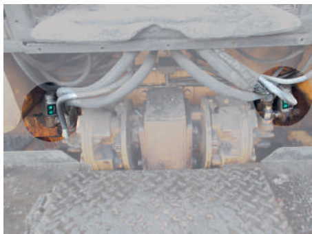
Mounting of AC700 on both conveyor belts
