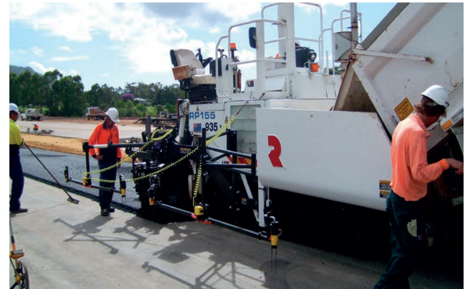
Averaging Beam with four grade sensors.
