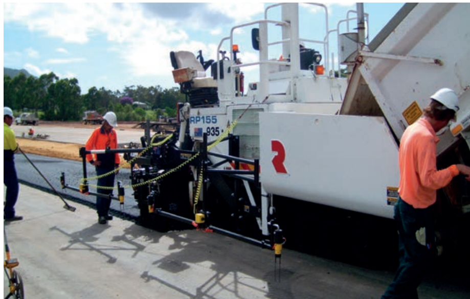
Averaging Beam with four grade sensors
